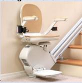
Used for internal building access Custom made to suit straight or curved/multiple flights of internal stairs Can be often operated by carer by using an infra-red remote control Often provided with safety features such as a retractable seat belt, safety sensors to prevent the seat from contacting obstructions on the steps, diagnostic information to show
